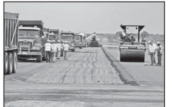
Teterboro's 6-24 Runway Gets Rehabilitated. November 2009
